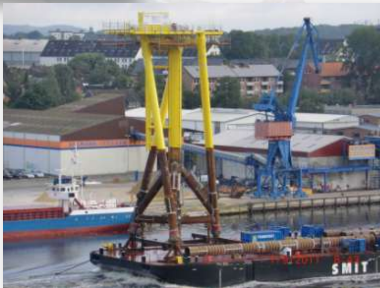
Figure 14 – Completed met mast with twisted jacket foundation (October 2011)
