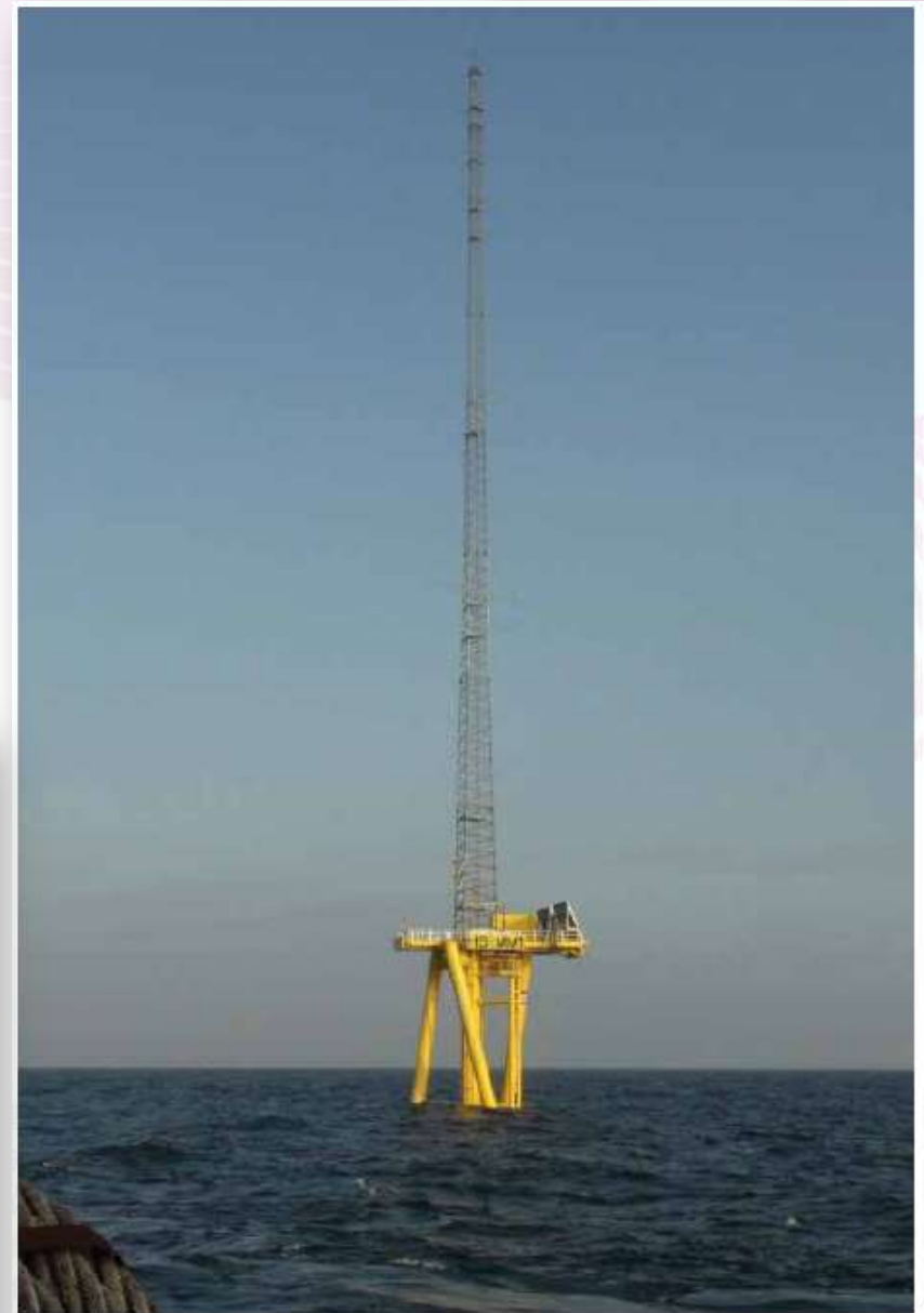
Figure 14 – Completed met mast with twisted jacket foundation (October 2011)
