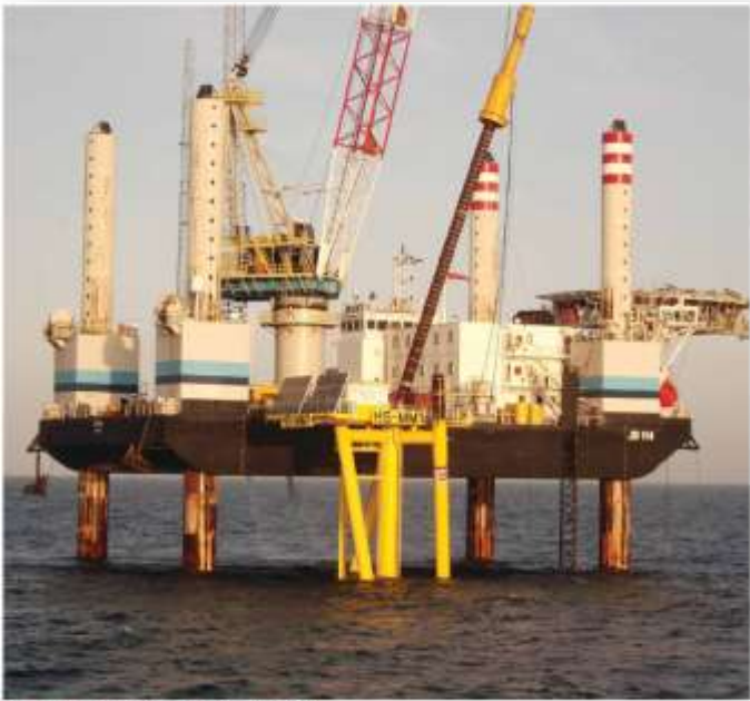
Figure 13 – Met mast installation (September 2011)
